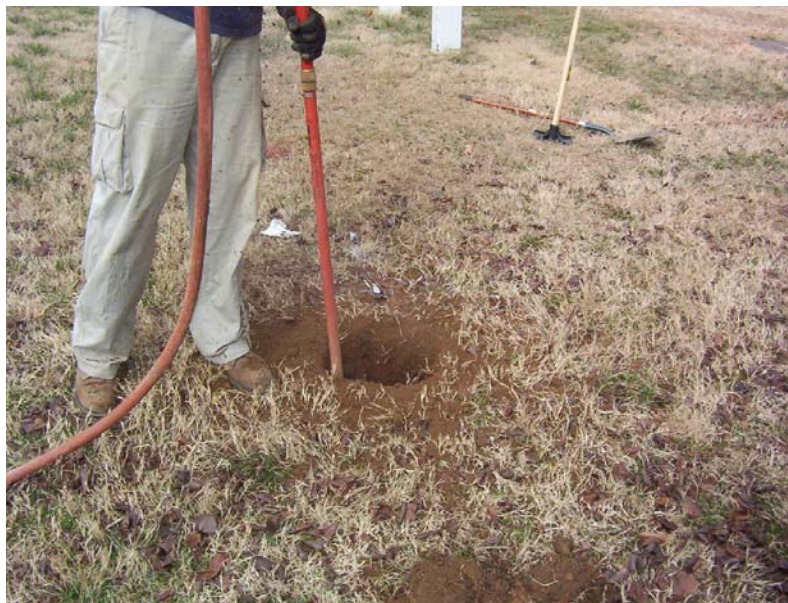
Figure 2.6 - Using an Air Knife (Photo courtesy of ATC Associates, Inc.)
